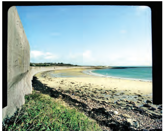
Anti-invasion wall around Longis Bay seen from a gun emplacement built into the wall
